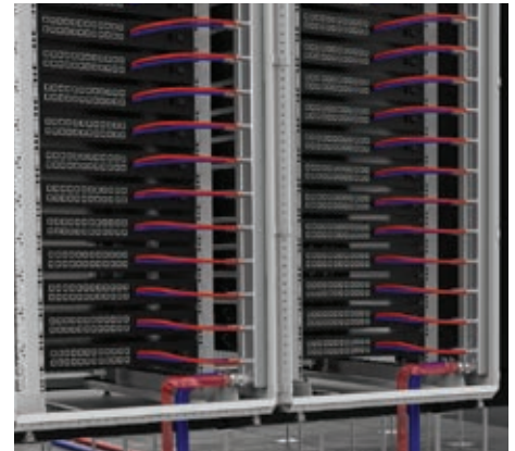
Rack manifold to manage liquid distribution
