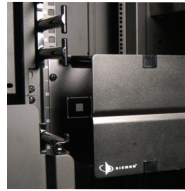
150mm (6 in.) of clearance between doors and frame
